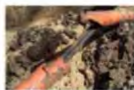
Utilities damaged by backhoe
