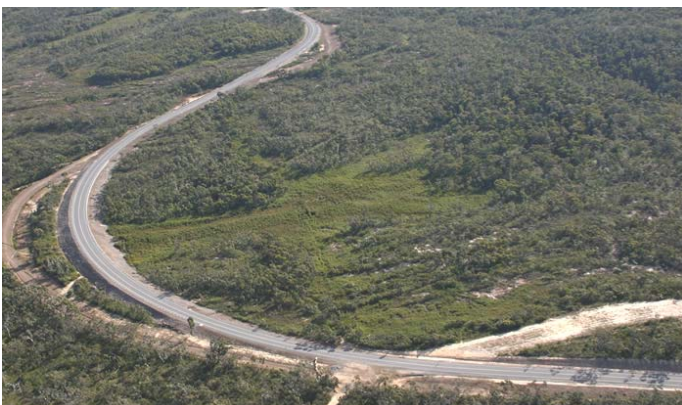
Completed work at Morton Park boundary
