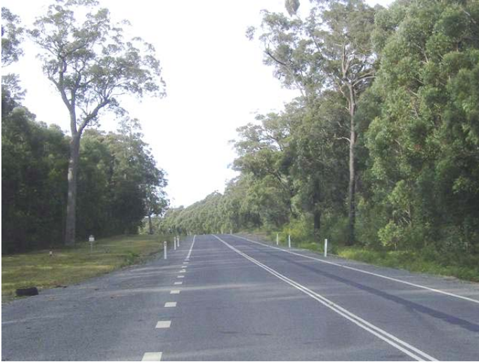
Completed work west of Turpentine Road
