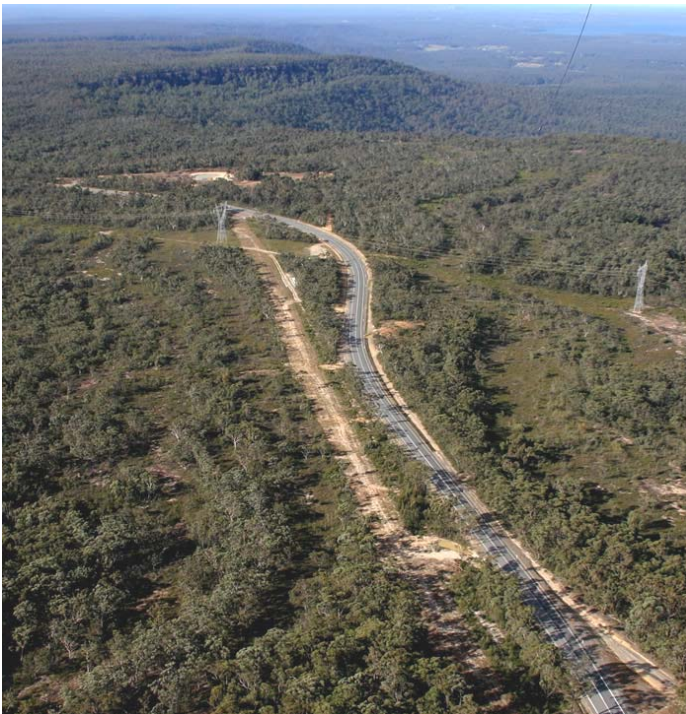
Completed work at Georges Yard
